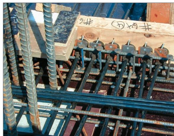
Studrails eliminate the need for hairpin reinforcement at tendon end locations easing reinforcement congestion.
