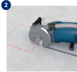
2 Cut the pattern using a saw depth of 1.5 inches.
