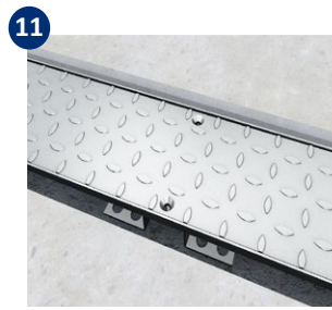
11 Attach the channel covers
