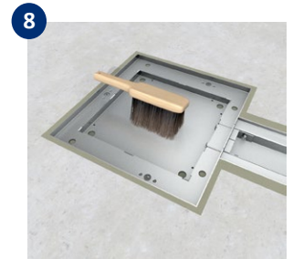
8 Clear all contaminants from the WCPS housing and channel.
